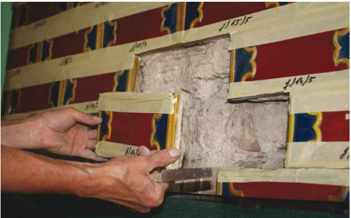
6. The numbered tiles during their removal
