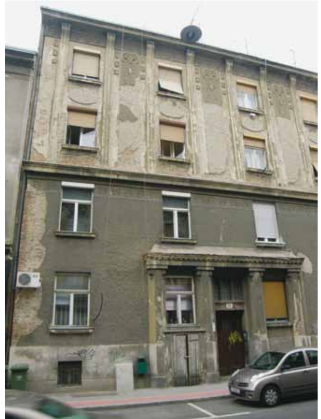
9. 80 Palmotićeva Street: Façade before the restoration
