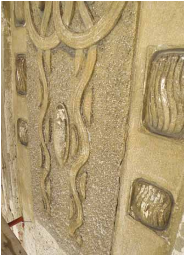
10. 80 Palmotićeva Street: Original stucco elements on the façade before the restoration
