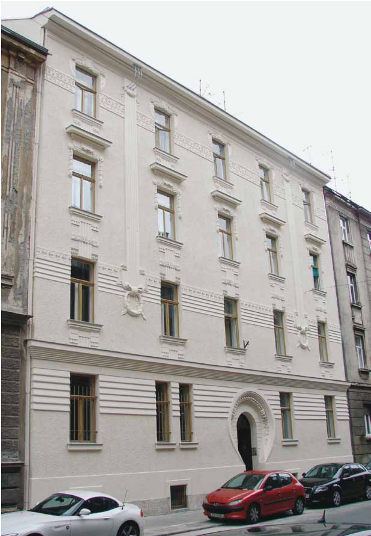
1. 20 Đorđićeva Street: Façade after the restoration
