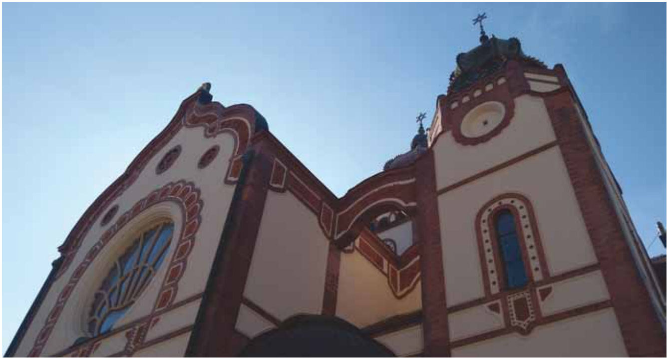
3. Northwest façade, restored in 1991
