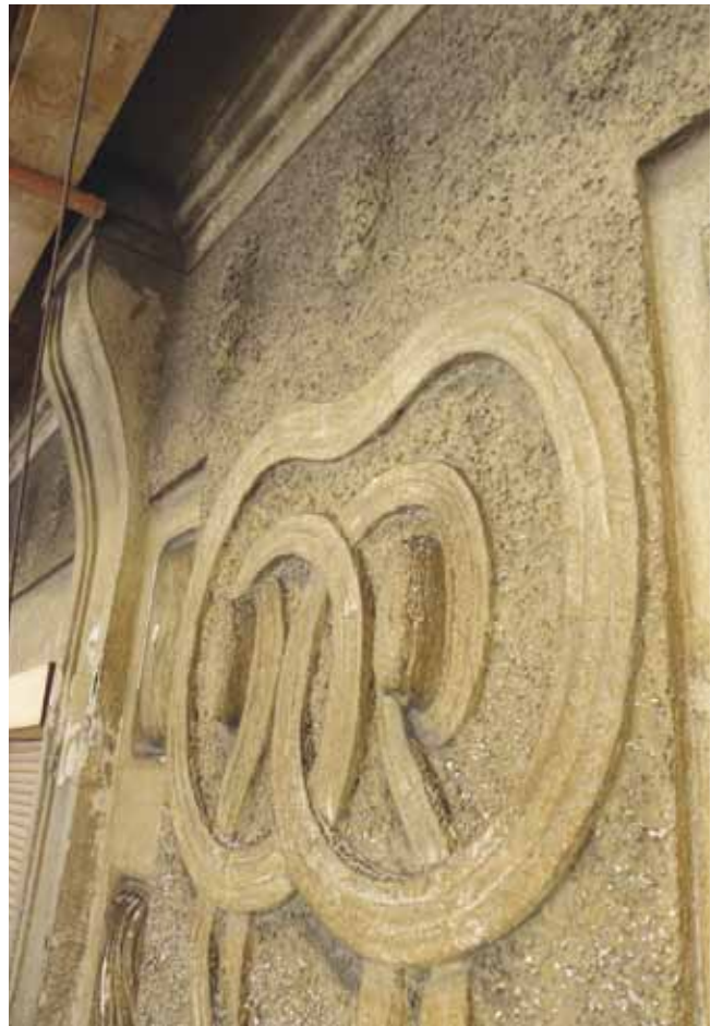
11. 80 Palmotićeva Street: Original stucco elements on the façade before the restoration
