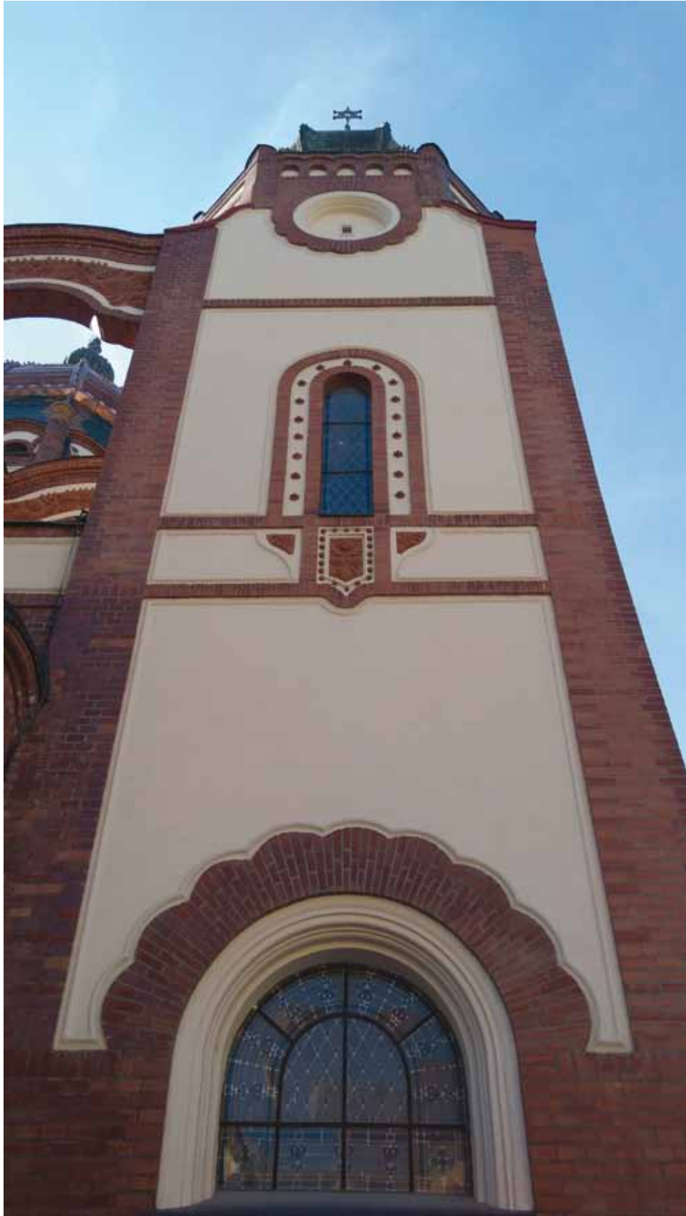
2. Northwest tower, restored in 1991
