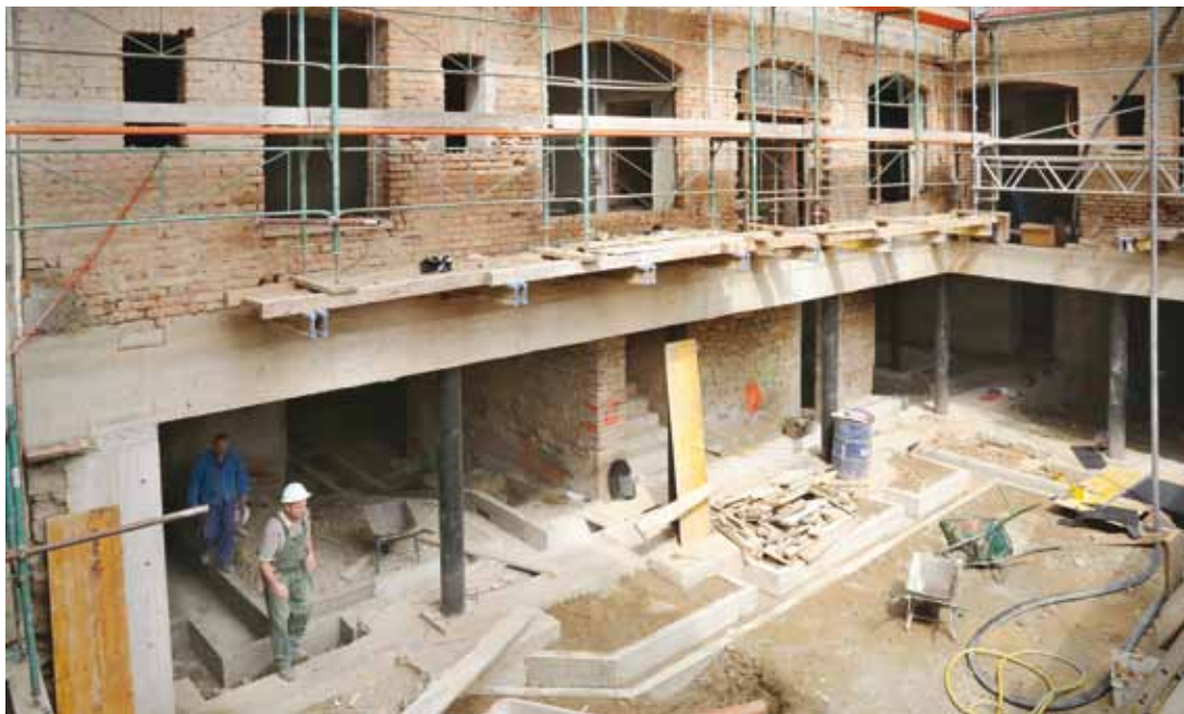
8. The entire basement level has been deepened and extended in order to incorporate the courtyard
