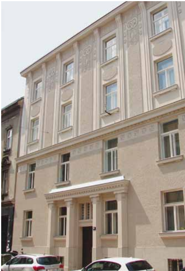
8. 80 Palmotićeva Street: Façade after the restoration
